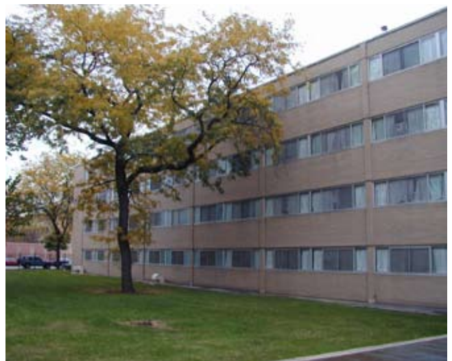
McCormick Student Residence
